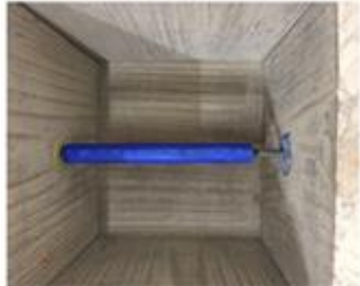
c) Hose used as bond breaker.
